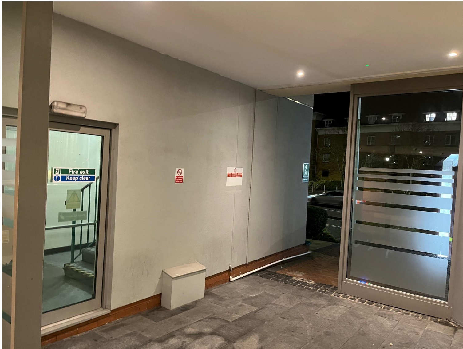
Photo 5 – Former Smoking Area
